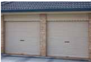
Examples of not approved garage doors
